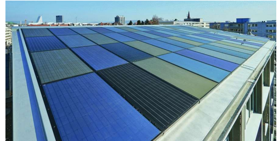
Kohlesilo CH-Basel, Solvatec AG
