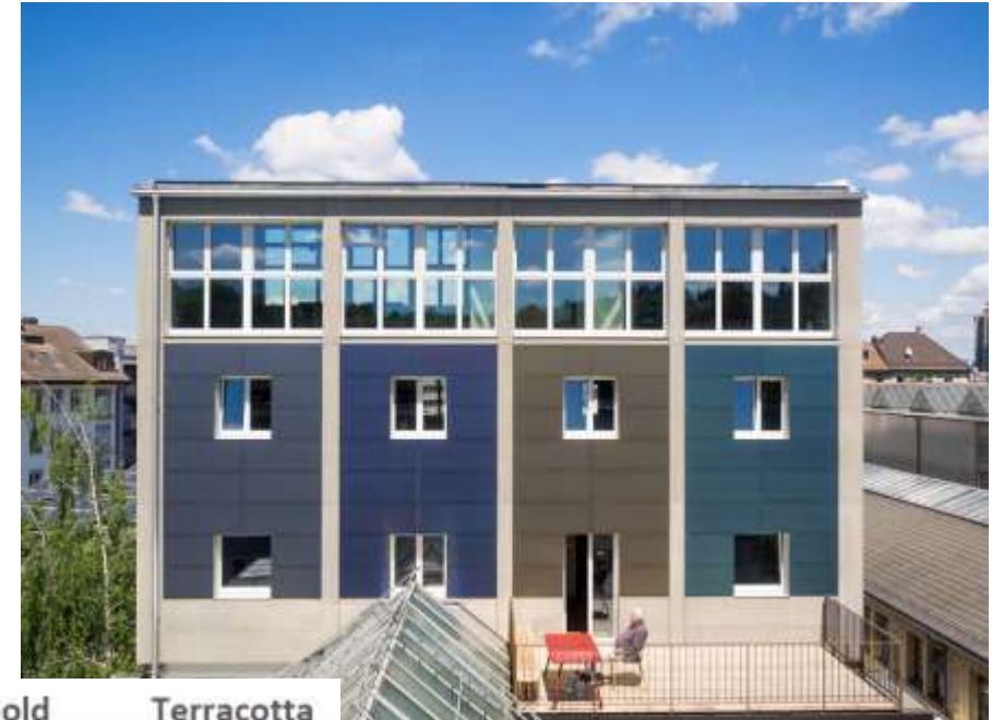
Kohlesilo CH-Basel, Solvatec AG
