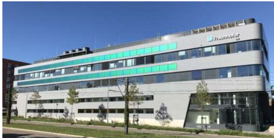
Fraunhofer ISE, Freiburg
